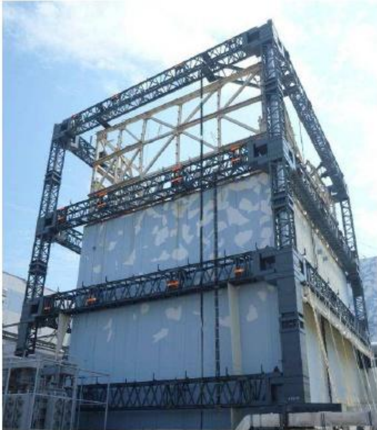
Sep. 9: Completion of steel-frame work (northwest side)
