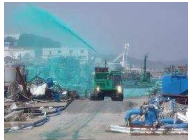
Dispersion of inhibitors around buildings of Units 1 to 4 by crawler dump
